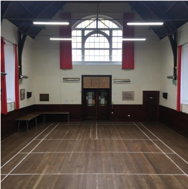
Figure 2: Town Hall Main Room from stage
