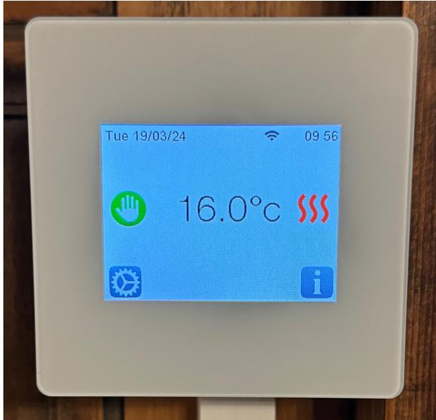
7. The room temperature will start to rise. Expect by 4-5 degrees Celsius an hour, until the target temperature is reached. Once at target temperature the thermostat will automatically turn off the heaters (red wavy lines disappear) and then turn them on again as required if the temperature drops below target.
