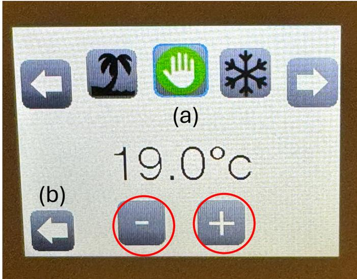
4. Scroll through the modes using the white arrows until 'Manual' mode (hand symbol) is highlighted in blue (a). You can use the + and – buttons to change the desired target temperature at this point if you wish. When happy, touch the white arrow on the bottom left (b) to activate the mode.
