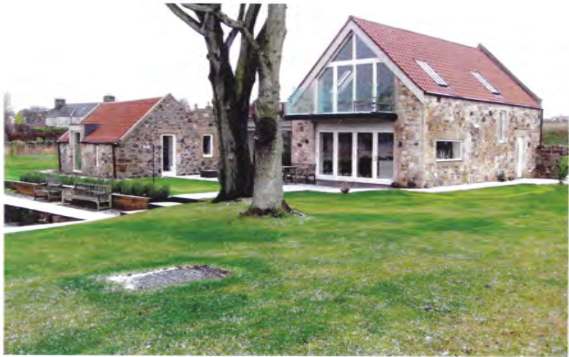
The completed renovations of Lochside Farm buildings
