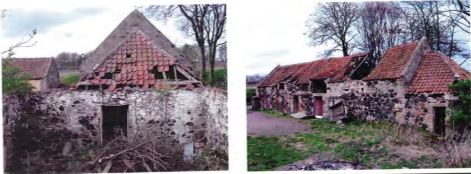
Lochside Farm buildings before renovation
