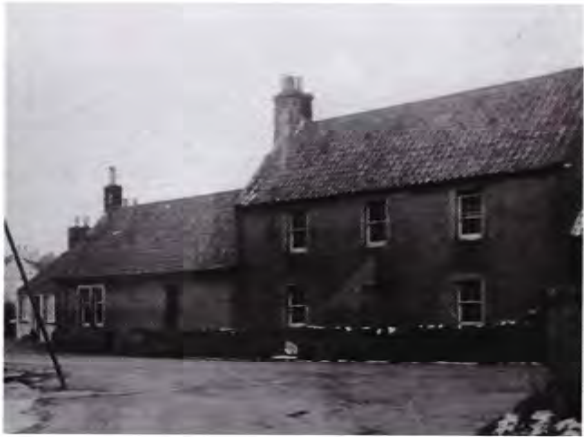
The old Farmhouse prior to restoration
